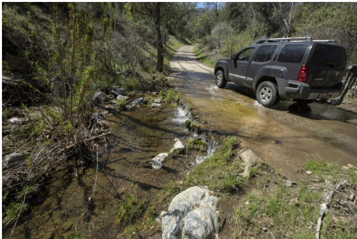
An SUV drives across Davy Brown Creek on a concrete apron, which will be removed and replaced with a bridge to allow fish passage. Brian van der Brug / Los Angeles Times
